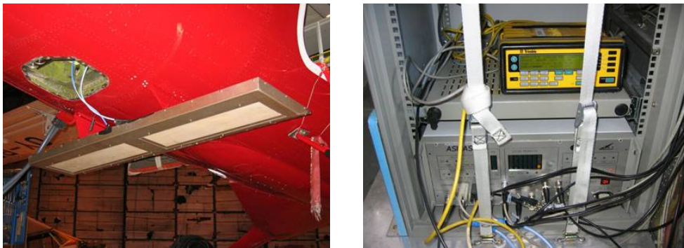
Photos of the ASIRAS installation.
